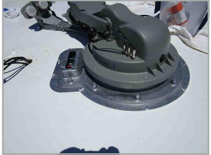
After you draw your location & drill the holes move the antenna away to apply dicor per the Trav'ler instruction, then set it back in place.
