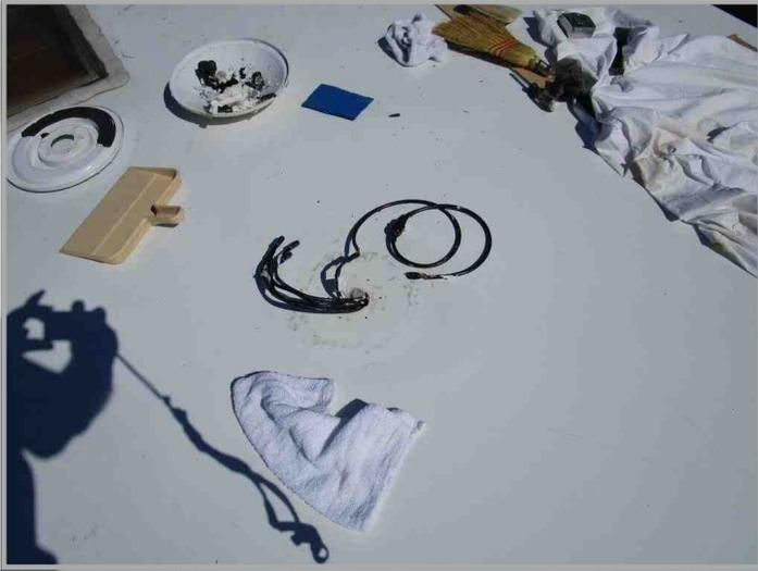
The picture shows the longer data cable and the 4 coax cables. This Trav'ler allows for only three coax cable connections.
