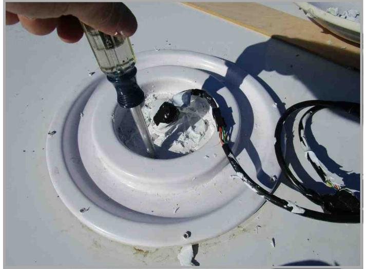
Now remove the 6 screws holding the bottom of the base. You have to dig out the dicor.
